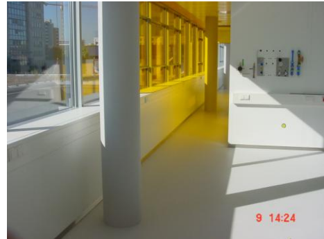
Construction of high school Laboratory area with parapet cladding
