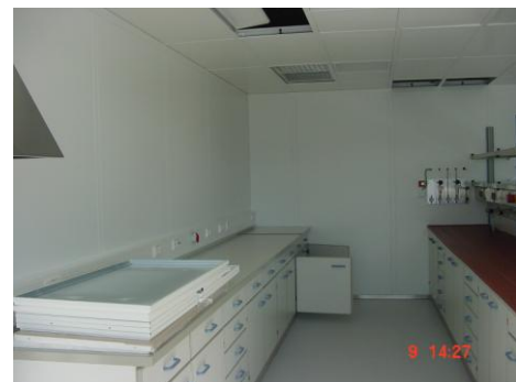
Subdivision of wall surface matching ceiling grid
