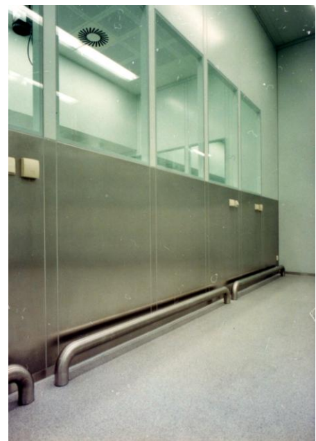
wall with glazing lower section in stainless steel
