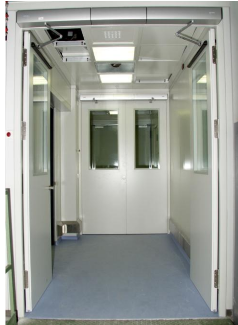
material pass-through 2-leaf swing door with door automation
